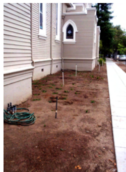
Homer Street side of the church
